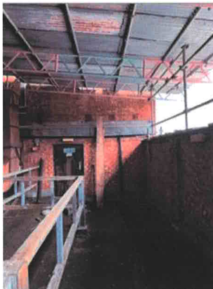
Plate No.2 Flat roof is of concrete construction over covered with asphalt. Drainage channel to the east side. Area enclosed both sides, 97 and 101 by 280mm soiled masonry wall approx 2.5mm high
